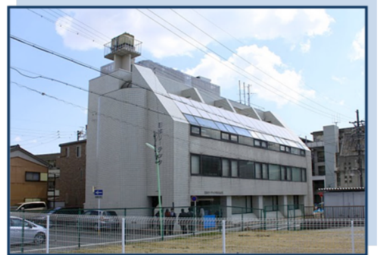
The building recently purchased for CBI ministry.
